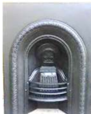
A Small Register Grate
